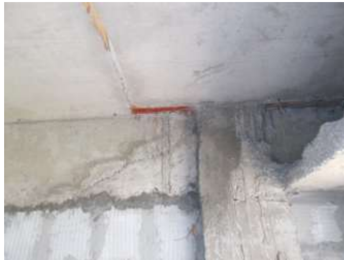
Fig ii Exposing Reinforcement & Honeycombing in Column-Beam Junction
