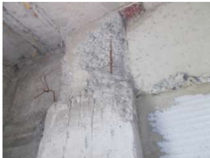
Fig iii Exposing Reinforcement in Column-Beam Junction
