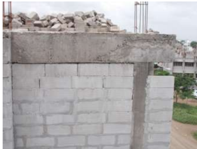
Fig v Honeycombing observing in Beam
