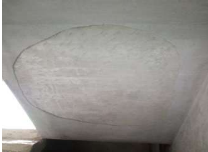
Fig iv Plaster Collapse at Staircase Flight
